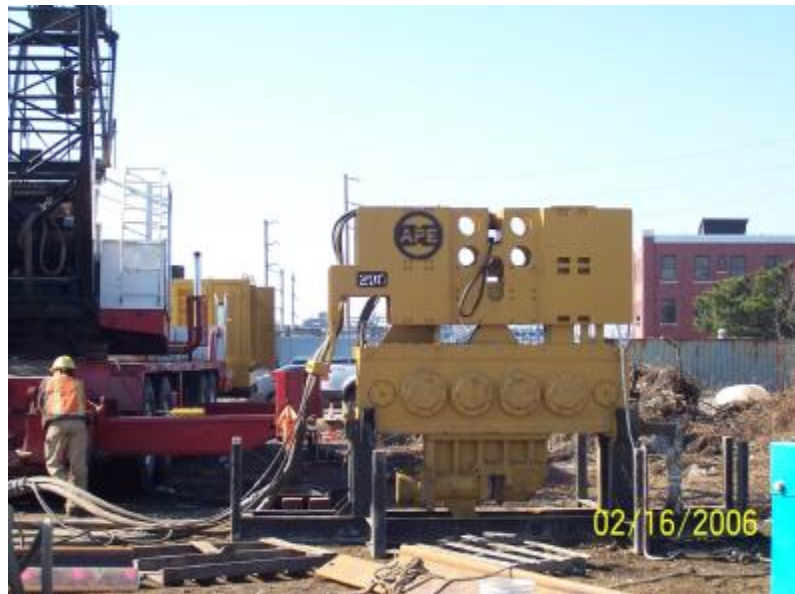
Photo 3: APE 200 Vibrator/Extractor
